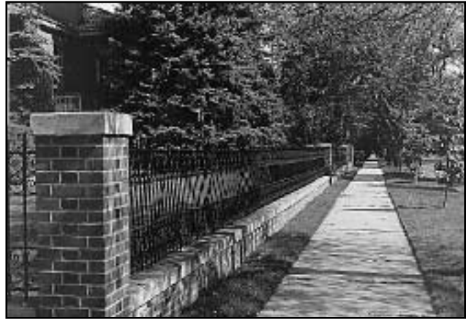
Front yard fences are typically constructed of brick and wrought iron or wrought iron. In all cases, views into the front yard maintain the sense of spaciousness.
